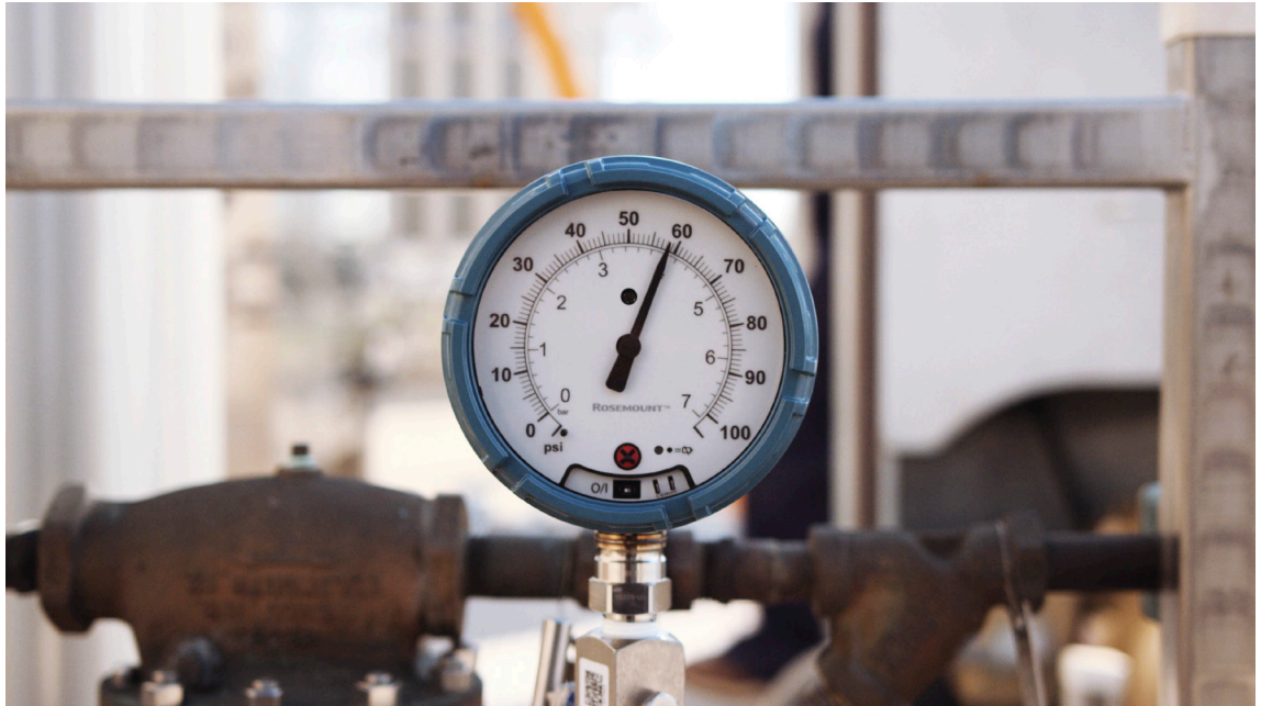
Figure 4.2: The Rosemount Wireless Pressure Gauge and Smart Pressure Gauge are identical except for the wireless capability.
